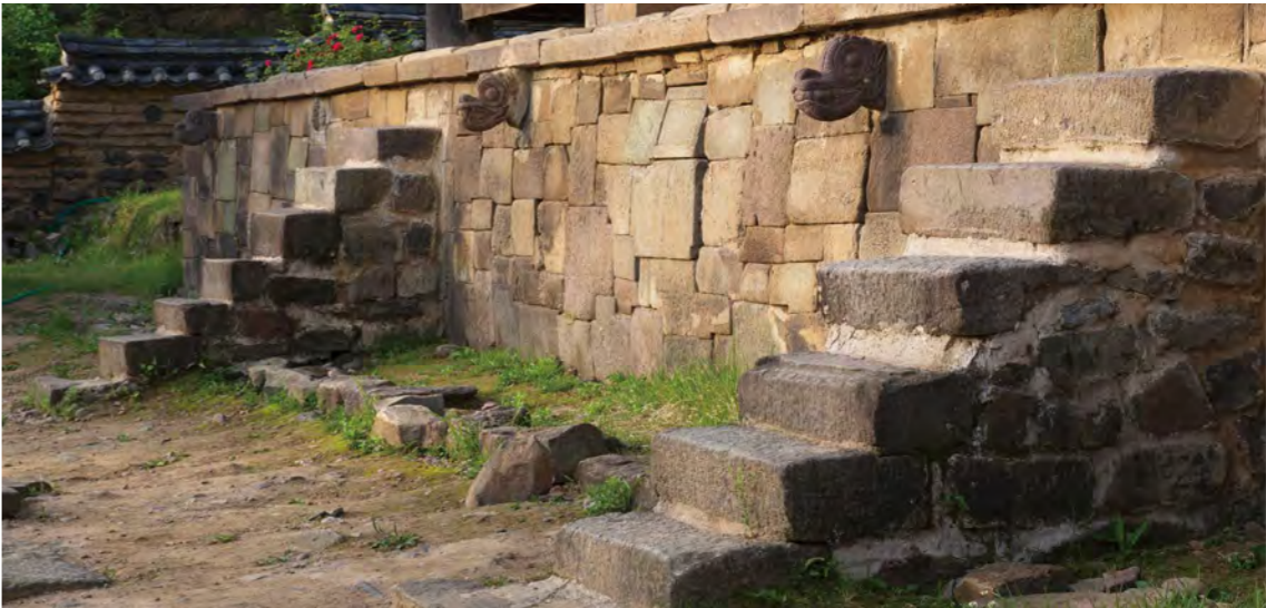
Figure 2-52. Stylobate and stairs of Jungjeongdang
